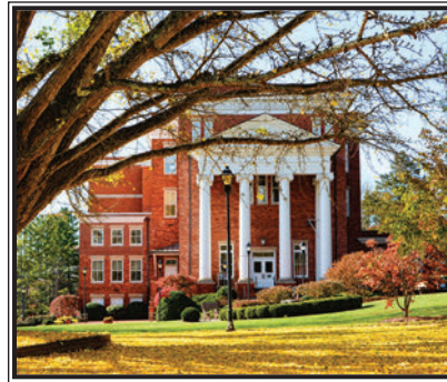
Lewisburg's Carnegie Hall is one of four buildings of the same name still in continuous use in the world.
